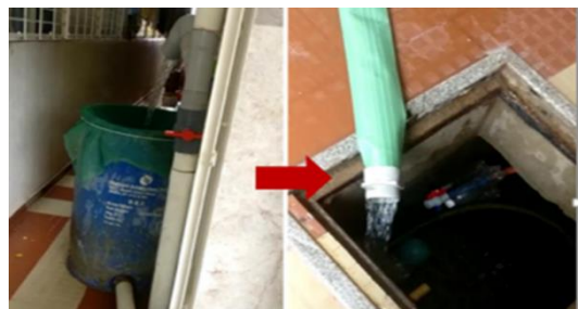
Figure 1: Effective and low cost RWH solution implemented in RWAs in Pavagada, Karnataka
